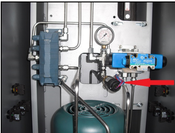
Figure 29- Pressure Switch Location
